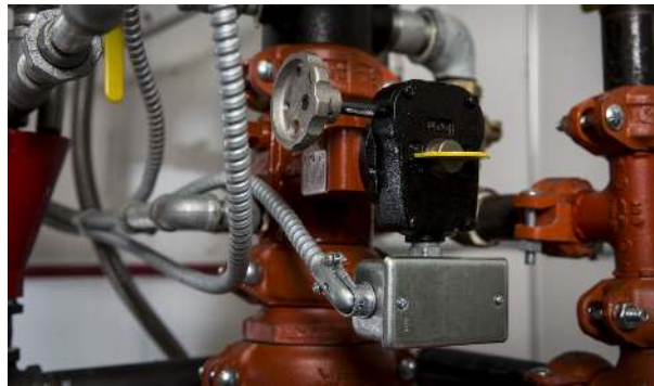
The number one reason for system failure is due to closed valves. This photograph is a clear example.
