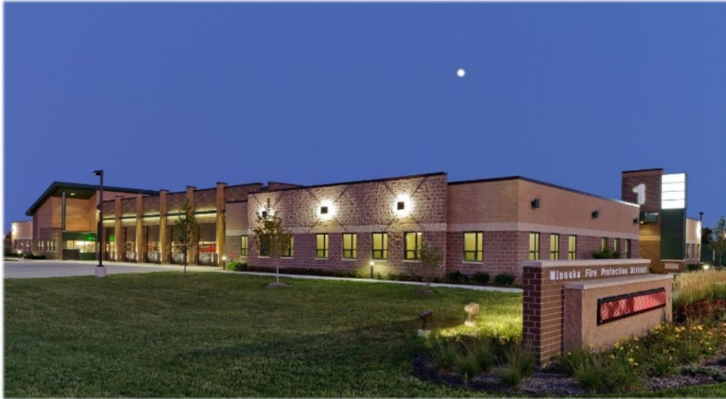
MINOOKA FIRE STATION #1- HEADQUARTERS
